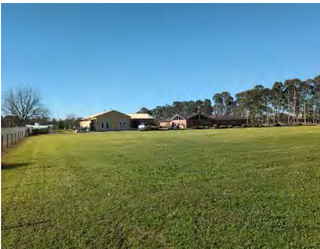
Figure 10. Buildings present and levelled landscape from north-west corner of project area.
